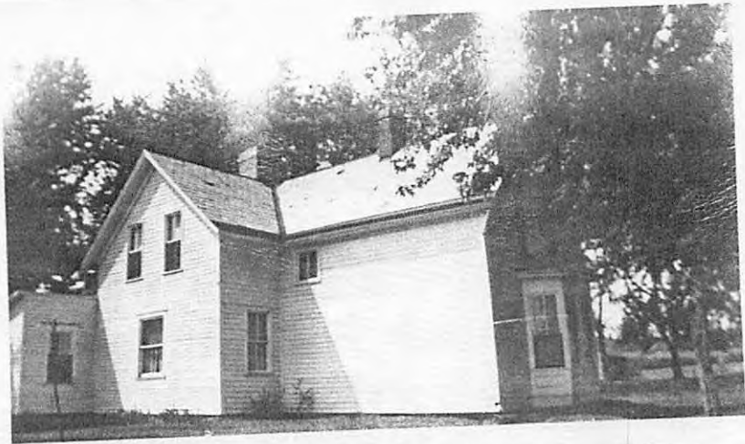
West side of house.
